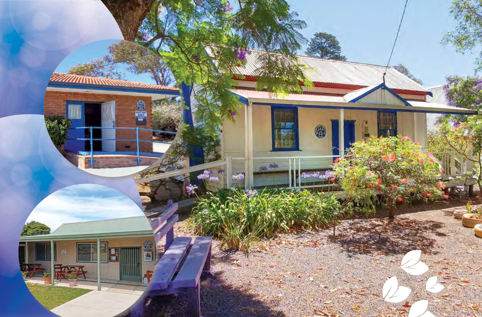
Left from top: Bluff Point and Hopetoun have had new air conditioning installed. Above: The Greenbushes Belles have repaired the verandahs of their charming cottage.
